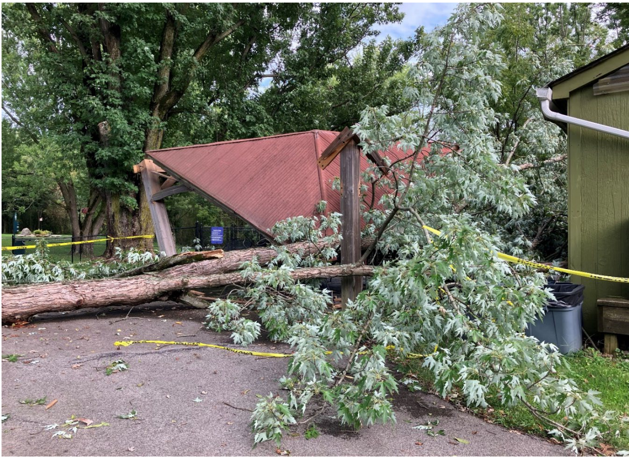
A violent thunderstorm on August 29 brought down a large tree limb in Sherwood Oaks Park, demolishing a covered sitting area near the garden shed.
