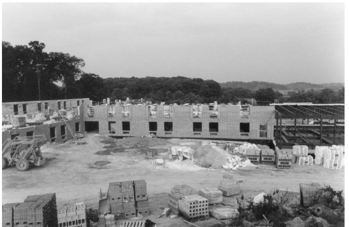
The Health Center walls are constructed. August 1981
