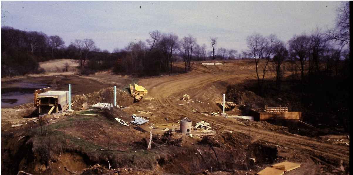
No gatehouse, no Norman Drive; just dirt, dirt and more dirt...April 1981
