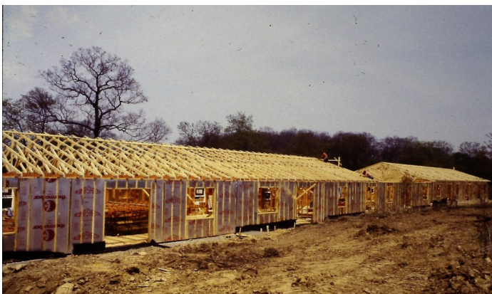
Patio home construction begins. May 1981
