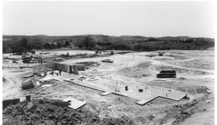
The foundation is poured for the Health Center. May 1981
