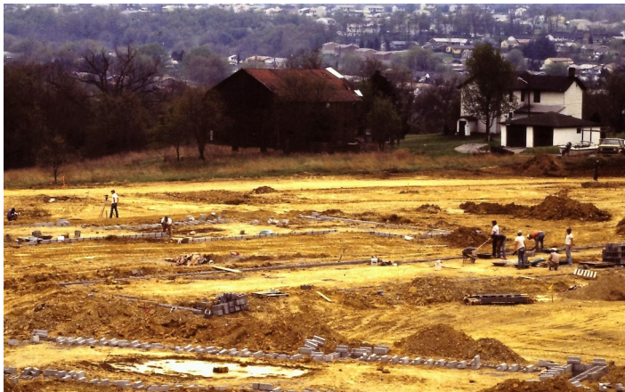
Workers prepare the land for construction. Note: Sherwood Oaks bought the Gettings farm (pictured at the top) in 1984. The barn was razed and the 90 yr. old farm house was used by the Fire Dept. for fire practice. The small white garage is still on campus, it is our Summerhouse. May 1981
