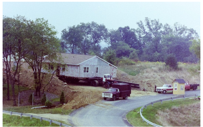
A small gatehouse was placed onto the paved roadway entering the community. The model homes/offices were placed in the area we now call "the Lake Parking Lot". Note: the paved roadway was not named Norman Drive as of this date. 1982
