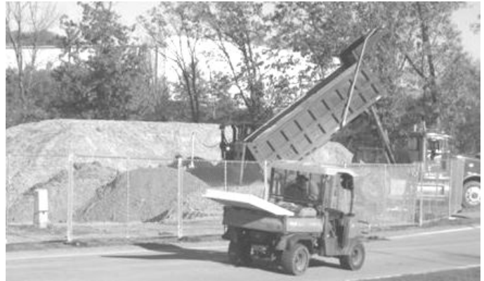
Dumping new soil for spreading by the bulldozer
