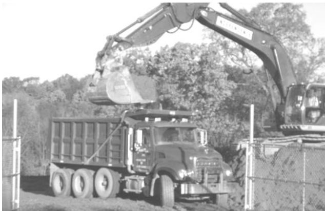
Removing unsuitable soil with a backhoe
