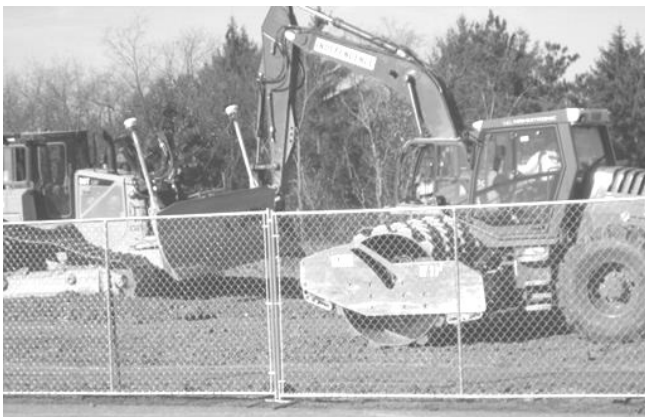
Bulldozer and sheeps-foot roller which is used for compacting fine grained soils.
